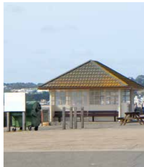
Figure 2.47 Victorian shelter along the promenade
