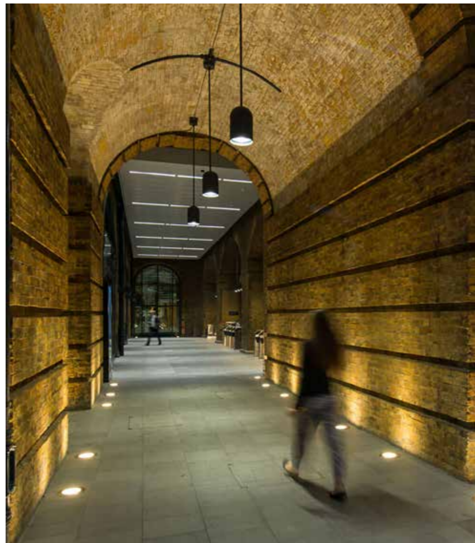
Figure 4.128 Inground uplighting and suspended lighting to arcades
