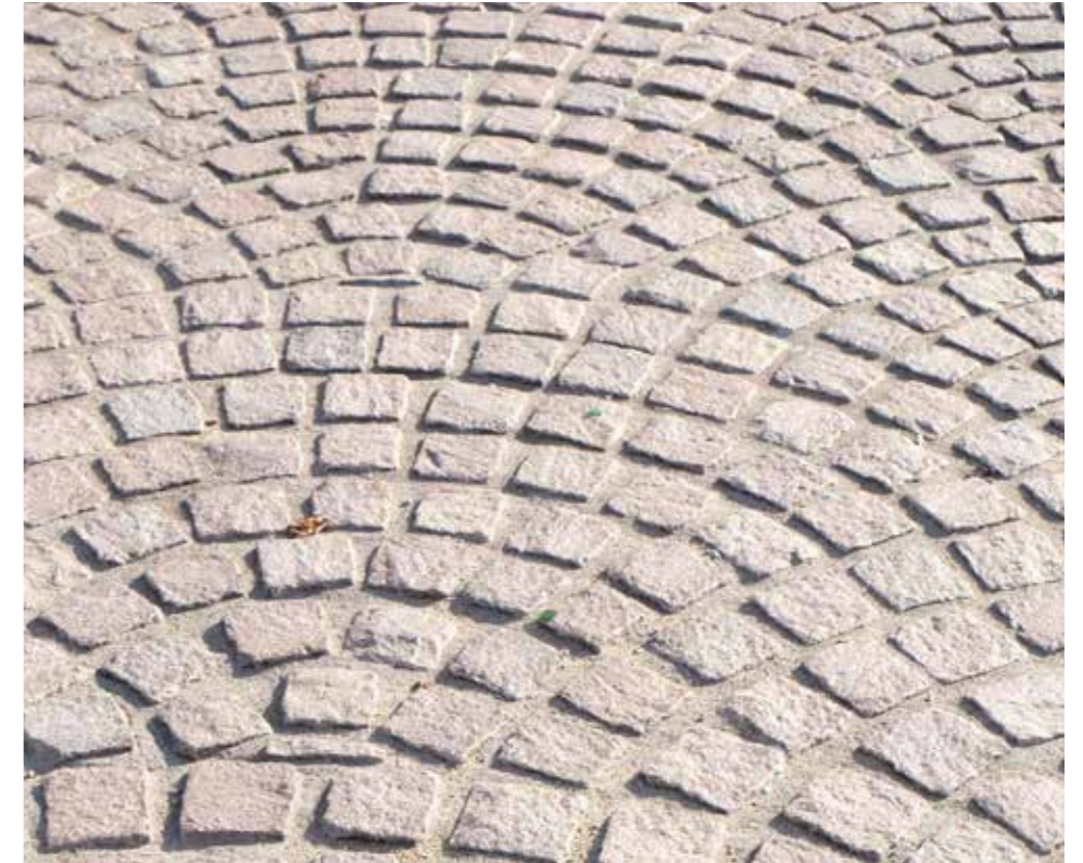
Figure 4.119 Fanned stone sett paving
