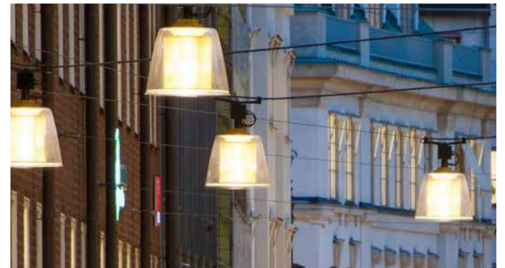
Figure 4.130 Catenary lighting to lanes
