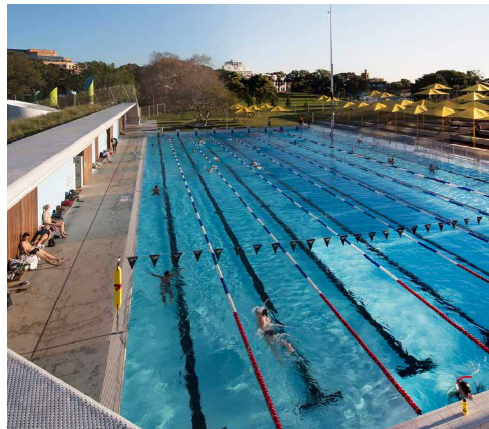
Figure 4.25 Lane swimming pool
