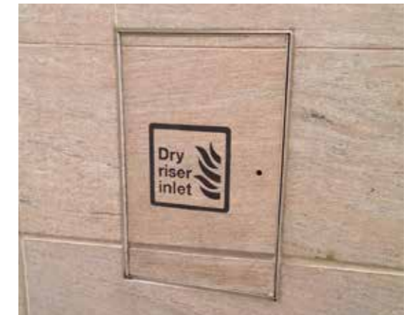
Figure 5.163 Example of a high quality coordination of façade with dry riser inlet
