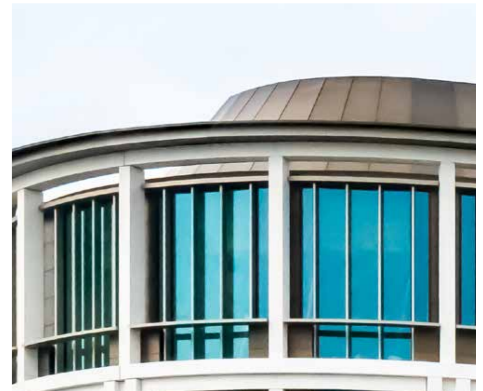
Figure 5.146 Roof top setback to minimise visual impact
