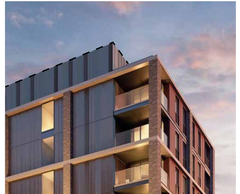
Figure 5.150 Façade over run to cover plant
