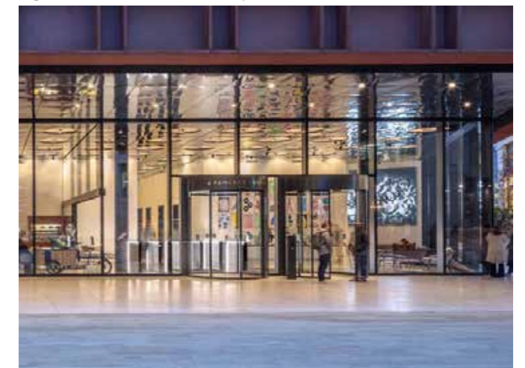
Figure 5.65 Commercial entrance integrated to façade
