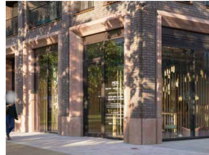
Figure 5.53 Frontage turning the corner
