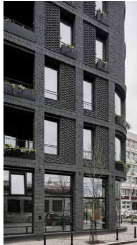
Figure 5.92 Example of windows with integrated window boxes
