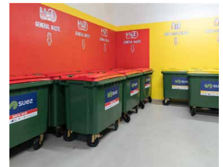
Figure 5.168 Example of basement bin store
