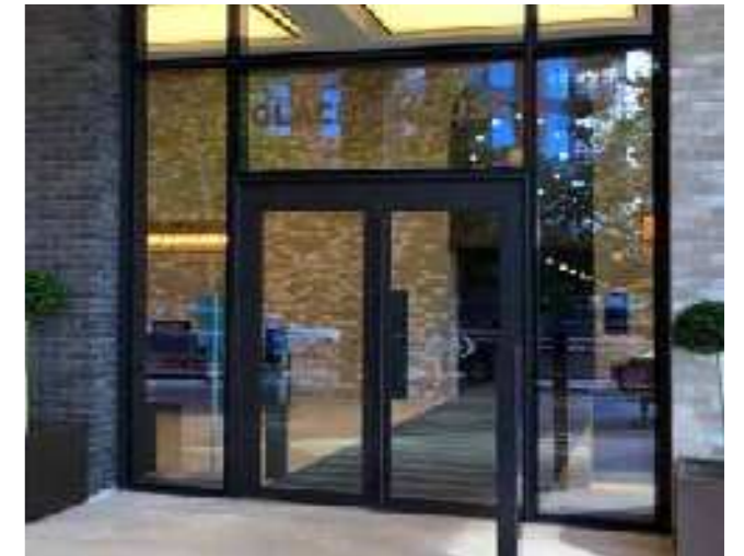
Figure 6.117 Example of a glazed residential lobby entrance
