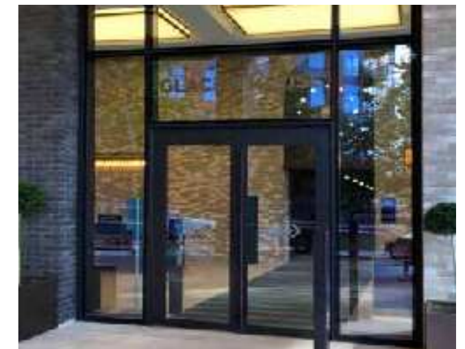
Figure 6.41 Example of a glazed residential lobby entrance
