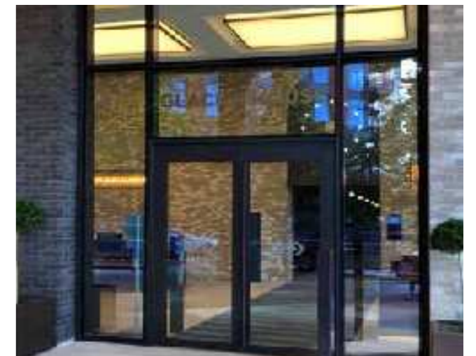
Figure 6.448 Example of a glazed residential lobby entrance
