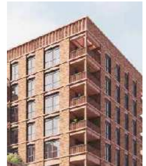
Figure 6.423 Example of inset corner balconies
