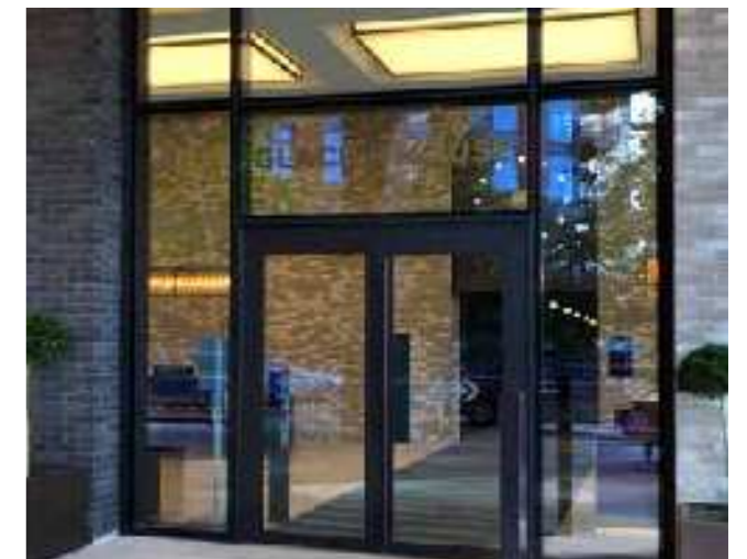
Figure 6.288 Example of a glazed residential lobby entrance
