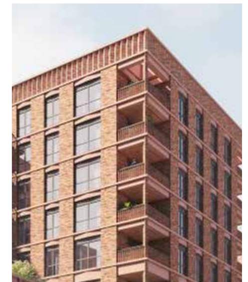
Figure 6.548 Example of inset balconies
