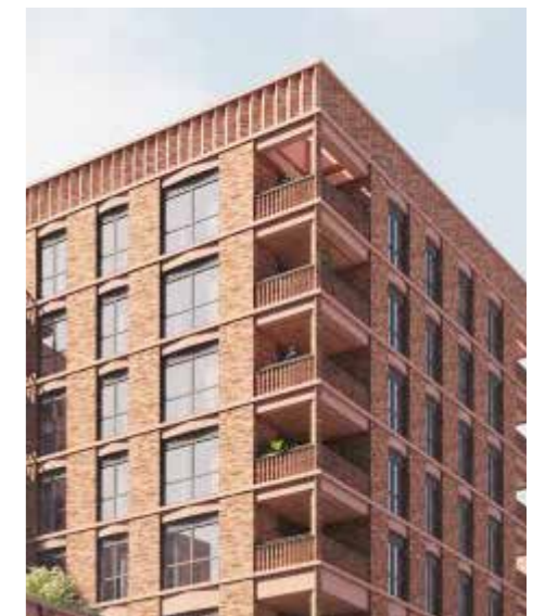
Figure 6.488 Example of inset balconies
