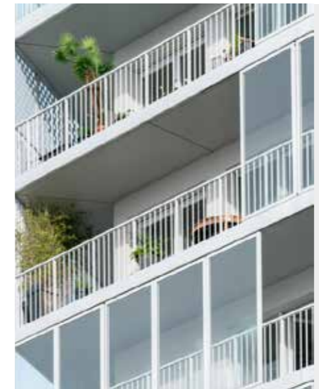
Figure 6.664 Example of inset balconies
