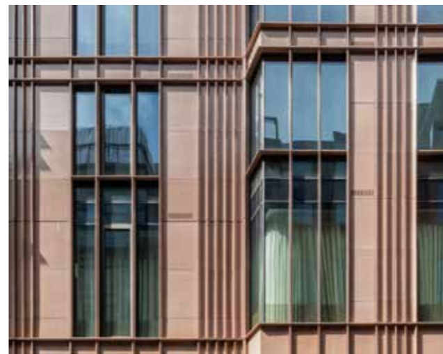
Figure 6.747 Acceptable high quality façade avoiding unrelieved stacks of glazing with integrated shading elements.
