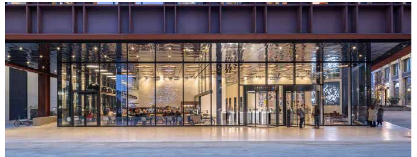
Figure 6.814 Example of separate entrance for office entrance and retail/food and beverage/cultural uses with glass partition between.
