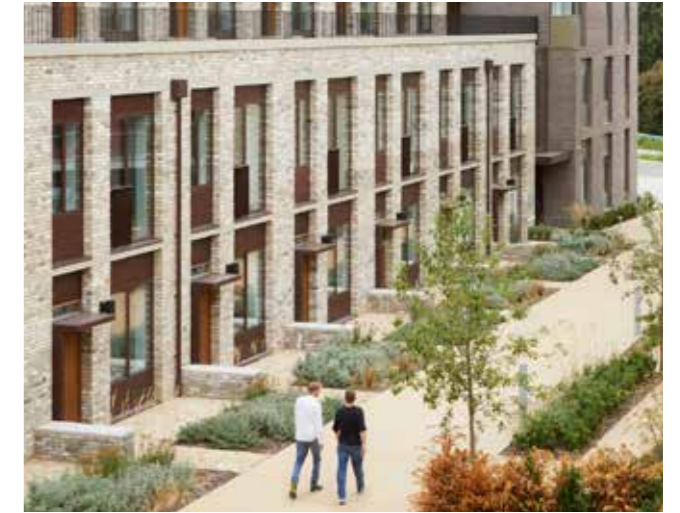
Figure 6.566 Example of a duplex residential entrances directly onto street
