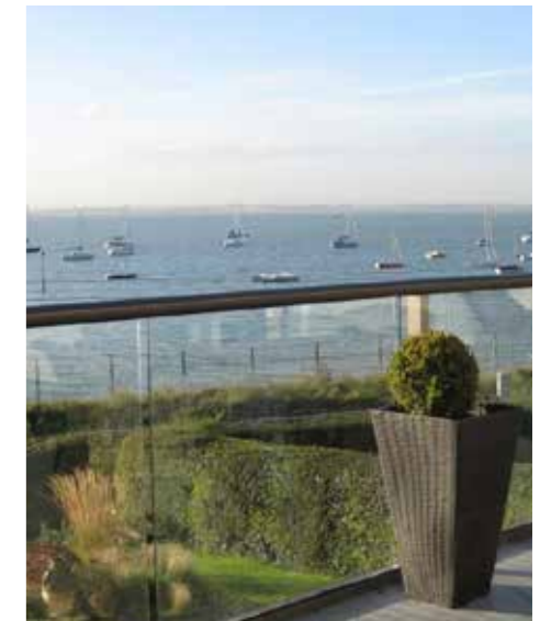
Figure 6.665 Example of 1.1m upstand
