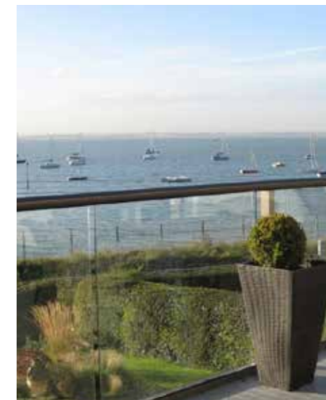
Figure 6.487 Example of 1.1m upstand
