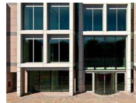
Figure 6.778 Concrete frame and painted steelwork
