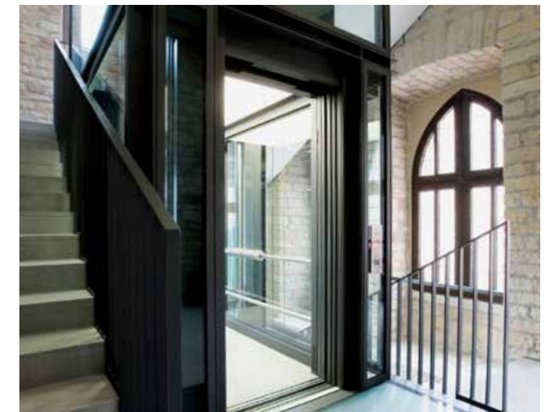
Figure 6.694 Illustrative example of integrated lift and stair to entrance circulation of residential block to accommodate level changes
