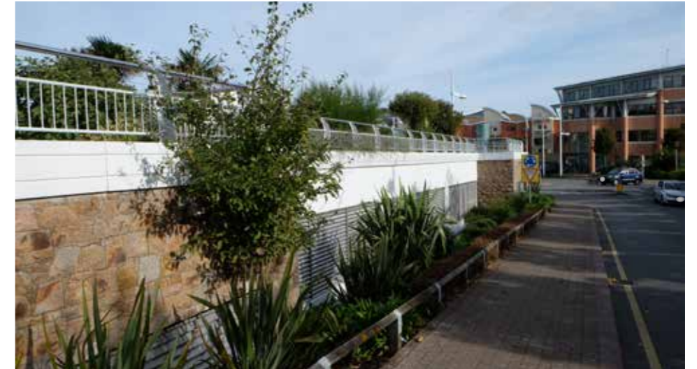
Figure 2.154 Level change to Marina Gardens basement along La Route du Port Elizabeth
