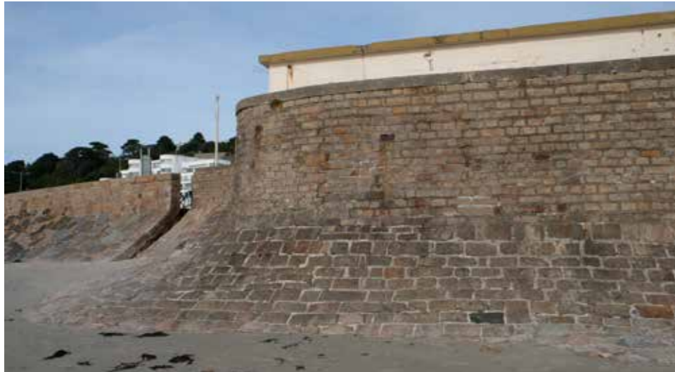
Figure 2.152 Seaward facing side of casemate with stair access
