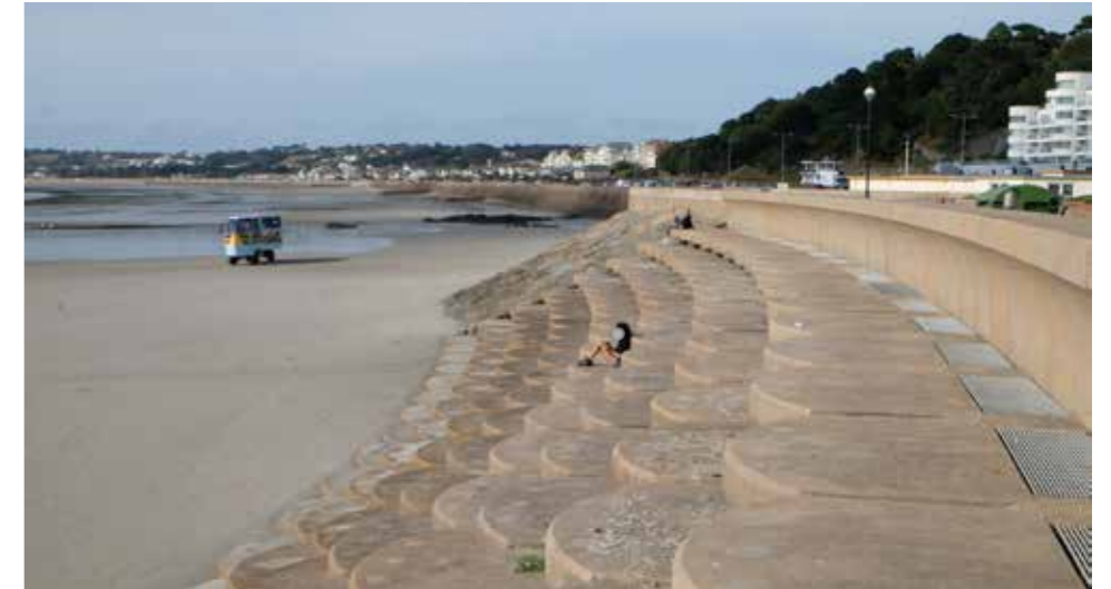
Figure 2.151 Stepped revetment down to beach level
