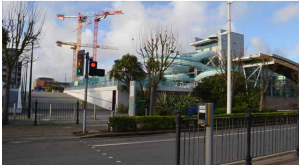
Figure 2.2 View from La Route du Port Elizabeth towards Aquasplash (1)
