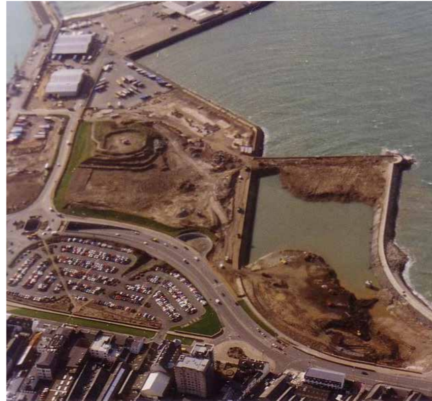
Figure 2.20 Image of the Site in 1995 showing the Esplanade, revetment area and the surface car park prior to redevelopment
