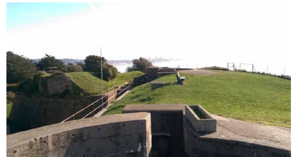
Figure 2.56 South Hill Battery and Gardens
