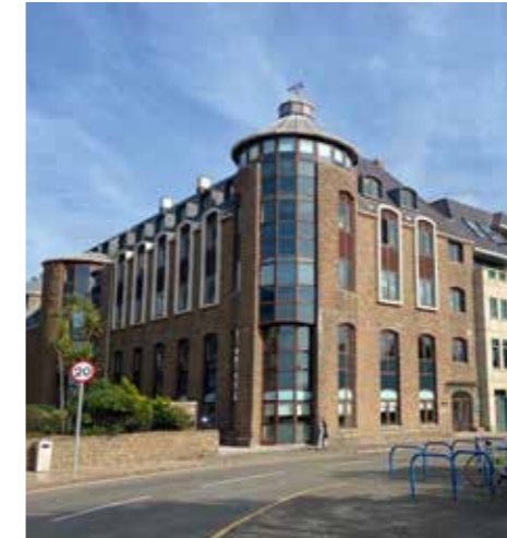
Figure 2.128 Site photos of the Esplanade
