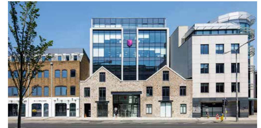
Figure 2.132 Site photos of the Esplanade
