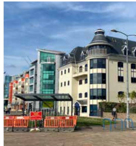
Figure 2.130 Site photos of the Esplanade
