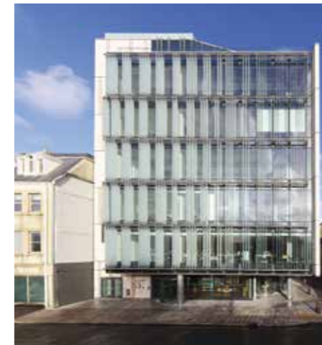
Figure 2.131 Site photos of the Esplanade
