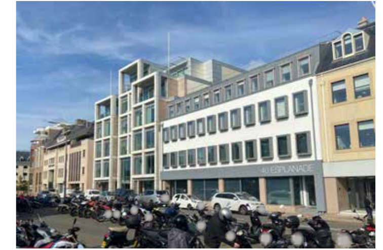
Figure 2.129 Site photos of the Esplanade
