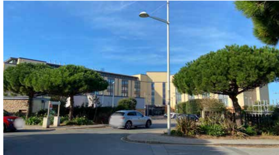
Figure 2.3 View from Rue de L'etau towards Radisson Blu hotel parking (4)
