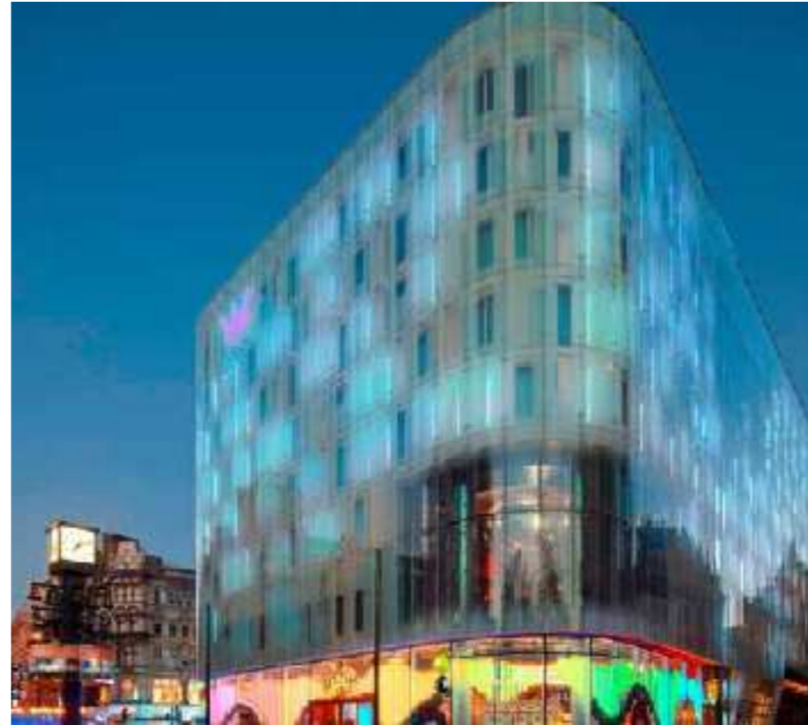
Figure 5.1104 London, UK Precedent: Turns the corner
