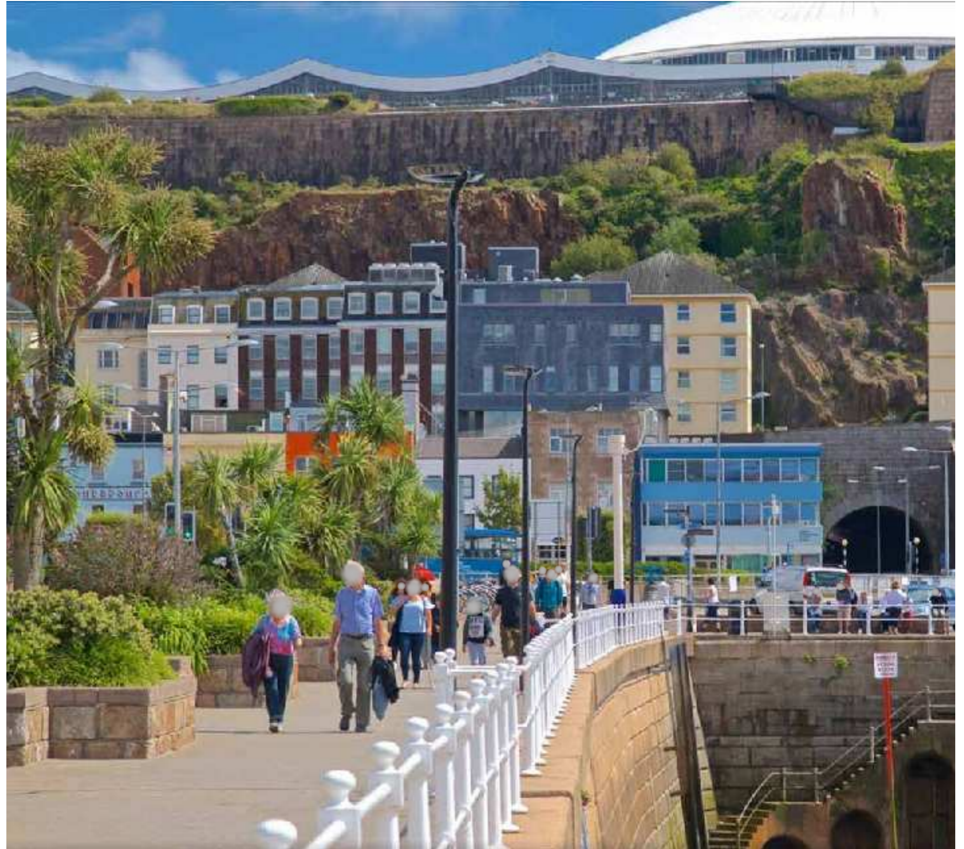
Figure 5.947 View of St Helier New North Quay looking towards Fort Regent
