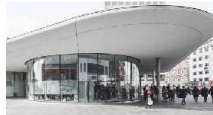
Figure 5.78 Public pavilion with sheltered waiting area
