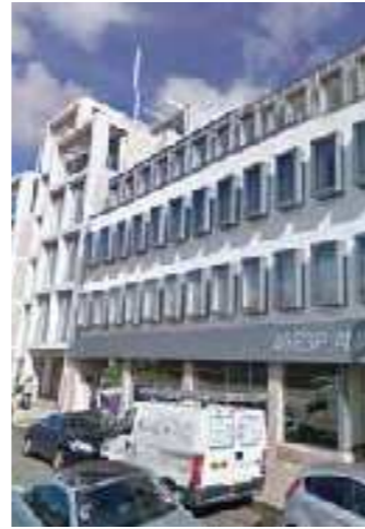
Figure 5.968 Frontage proportion at 40 Esplanade, Jersey
