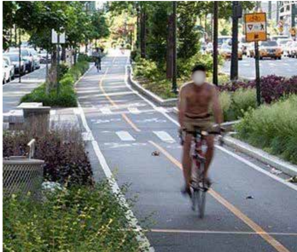
Figure 5.165 Planting used to separate the cyclist from pedestrians and vehicles
