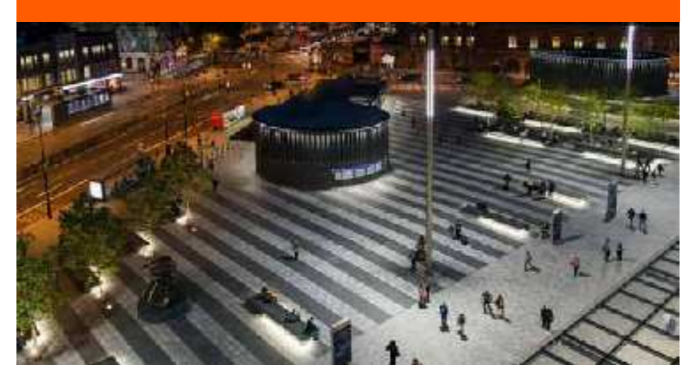
Figure 5.895 Pole mounted lighting to squares
