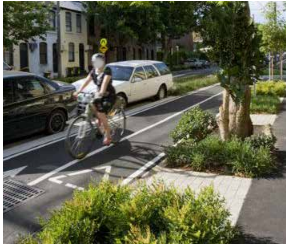
Figure 5.164 A dedicated cycleway protected by planting
