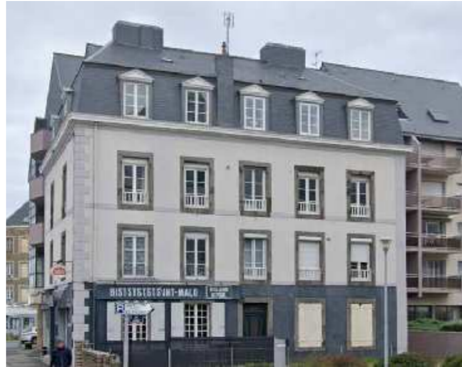
Figure 5.1041 Saint Malo historic building reference
