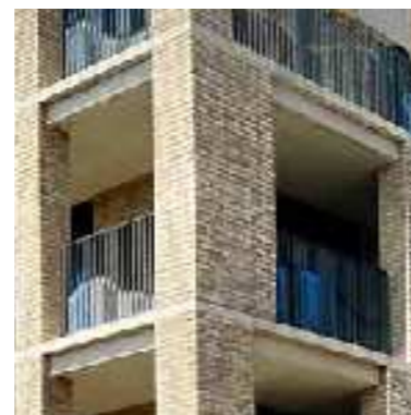
Figure 5.1030 Example of opened corner balcony treatment
