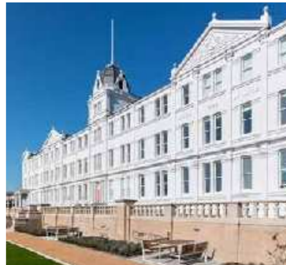
Figure 5.1080 Collage Gardens, Jersey: Fenestration proportions and cornice line in details
