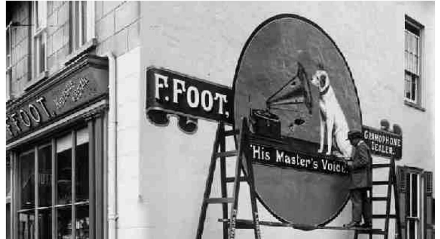
Figure 5.889 Historic photo of the HMV sign on Dumaresq Street
