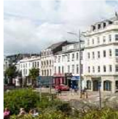
Figure 5.1017 Typical Jersey vertical façade division through treatments, and arrangements along the Esplanade
