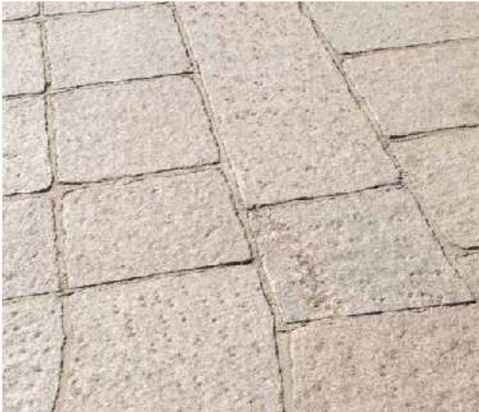
Figure 5.841 Hammered stone finishes and long stone pavers used to create edges
