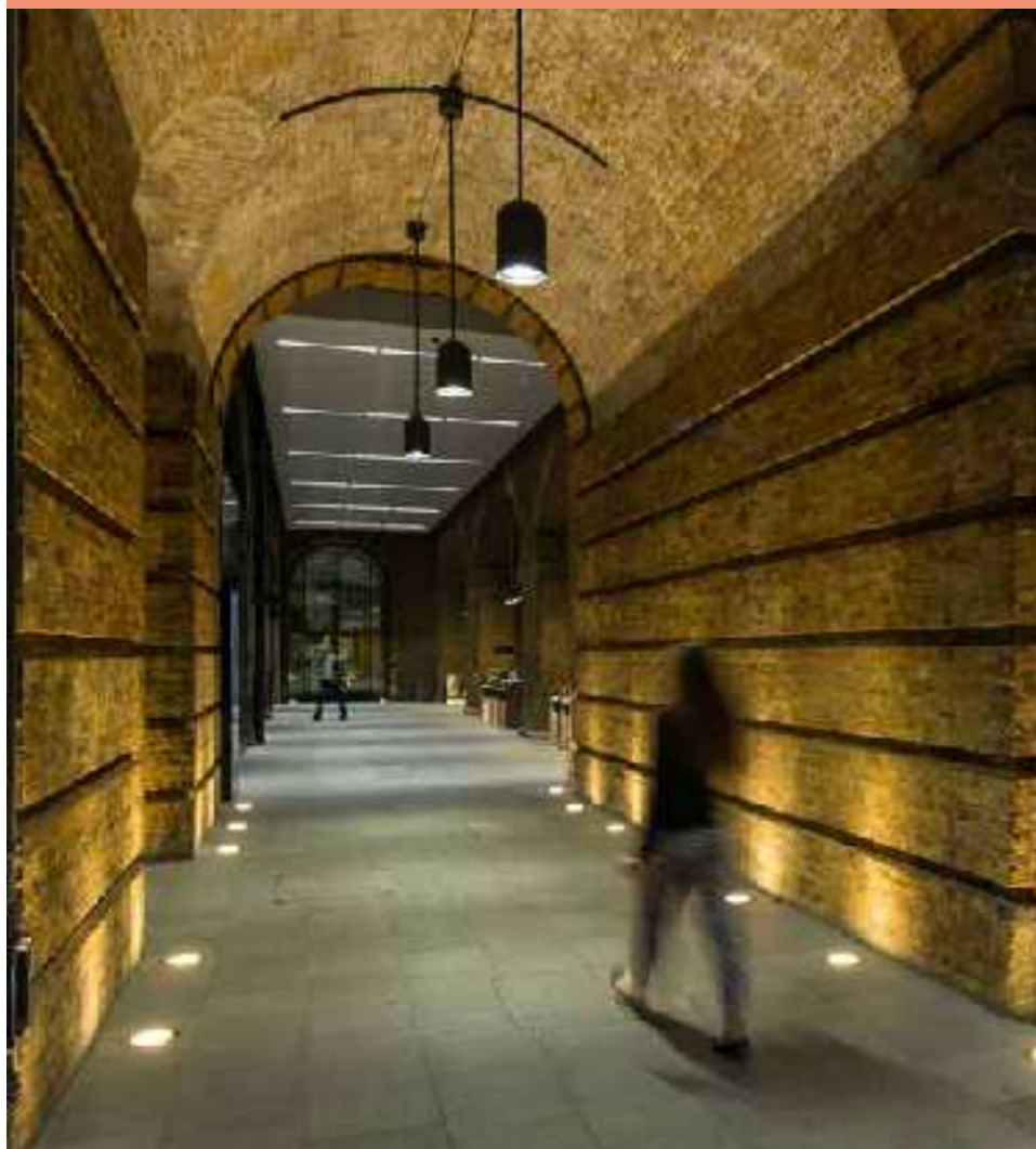
Figure 5.896 Inground uplighting and suspended lighting to arcades
