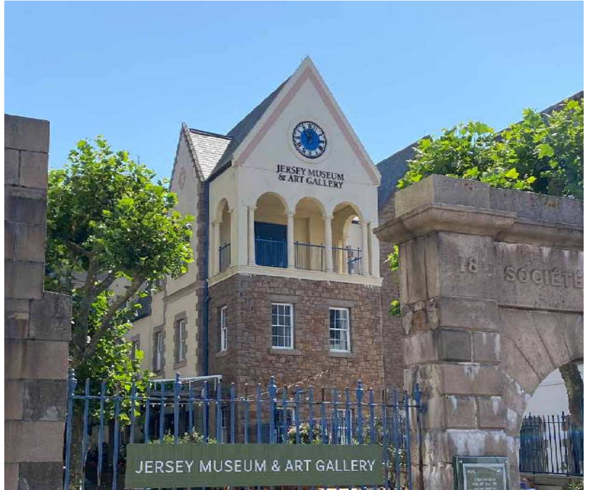
Figure 5.1040 Image of the Jersey Museum and Art Galley, an example of a distinctive building with its own identity
