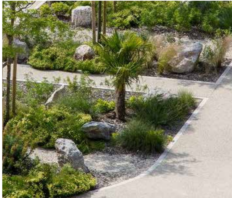
Figure 5.159 Wide bioswales with pedestrian routes through
