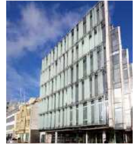
Figure 5.961 Modern example - Price Waterhouse Cooper building - louvres / façade treatment
