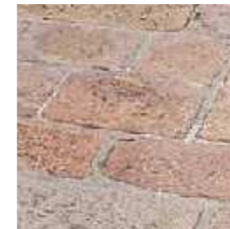
Figure 5.16 Local pink granite paving
