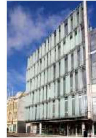
Figure 5.986 Price Waterhouse Cooper Building
