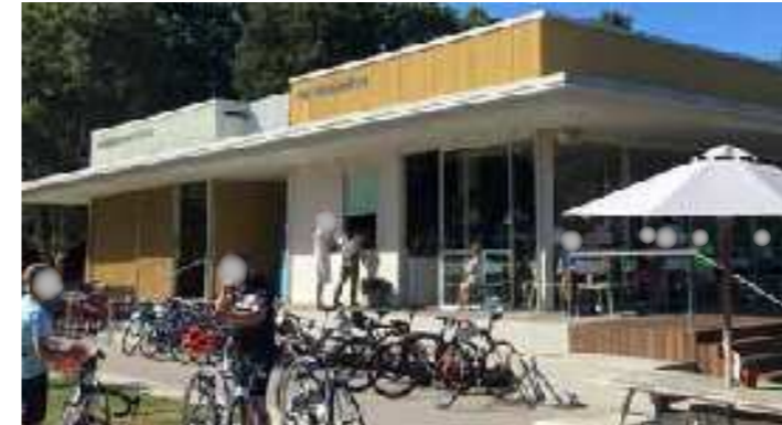
Figure 5.74 Cycle parking integrated with building
