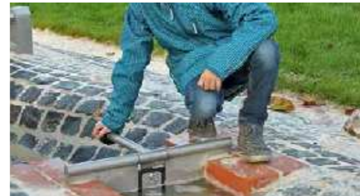
Figure 5.908 Water channelling and damming
