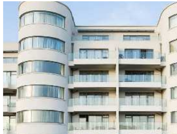
Figure 5.1060 St Helier precedent, St Aubin’s Road: Frontage proportion
