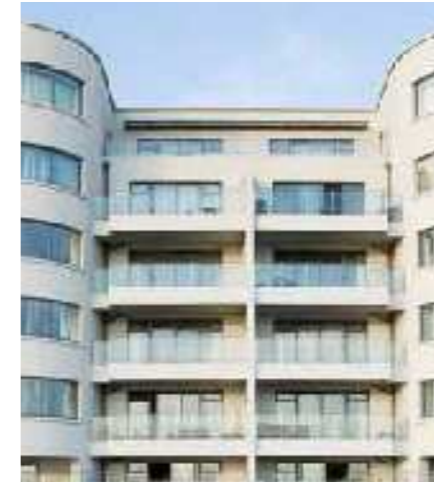
LOCAL and INTERNATIONAL INSPIRATION Figure 5.960 St Aubins Road
