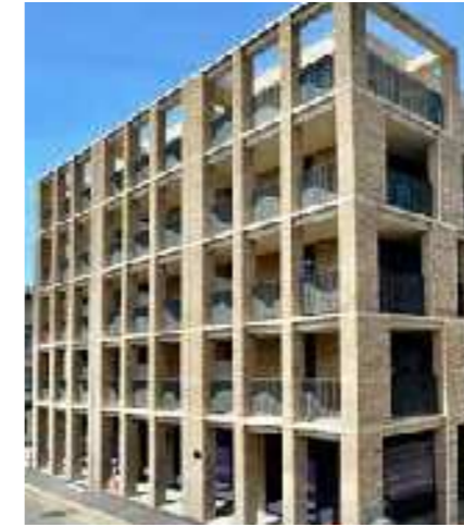
Figure 5.951 Ed Le Quesne House - inset balconies and detail in railings
