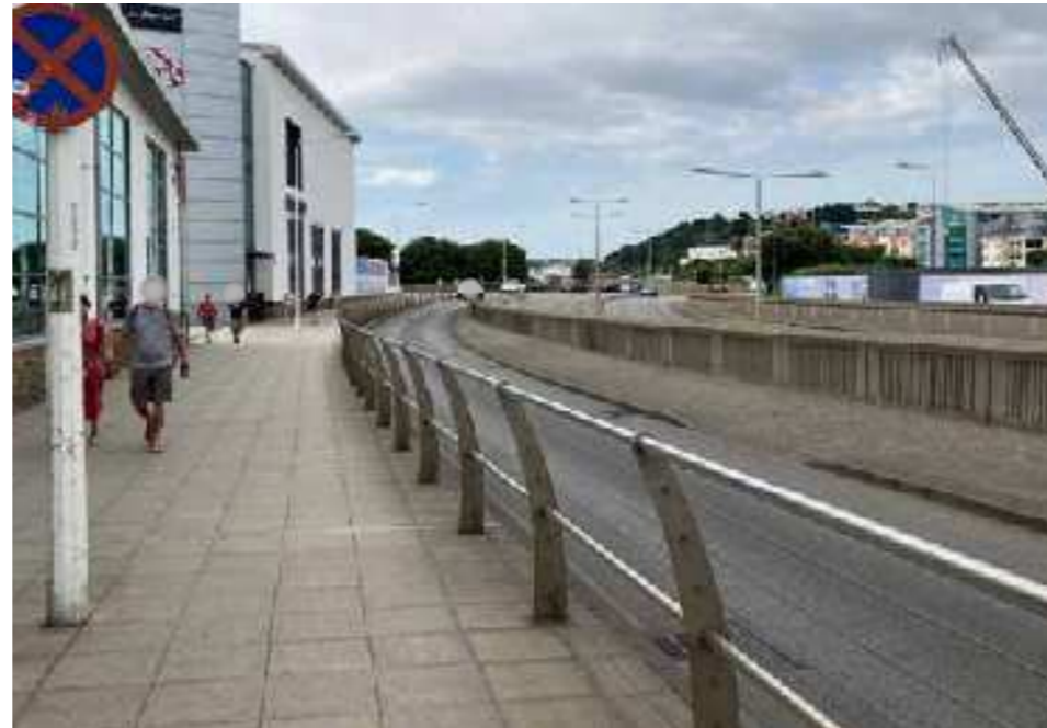
Figure 5.168 Viewpoint 1 looking north from Block F1 corner - existing condition
