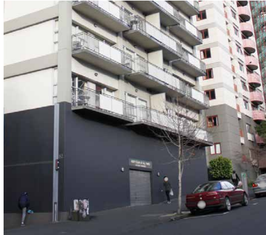
Figure 2.162 Blank facades at ground floor resulting in an inhospitable pedestrian environment
