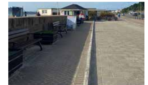
Figure 6.29 Kerbs along promenade
