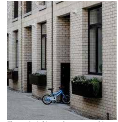
Figure 4.59 Clutter free street with no or private defensible zones interrupting the public realm. Possibility for window boxes
