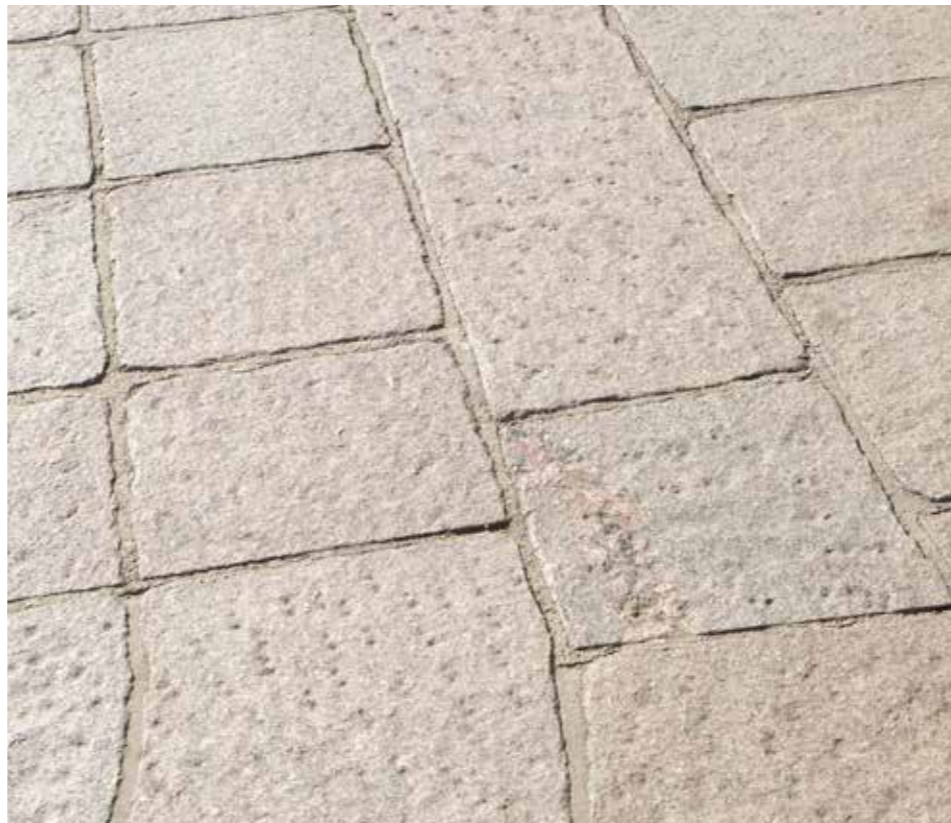
Figure 4.118 Sparrow pecked stone finishes and long stone pavers used to create edges
