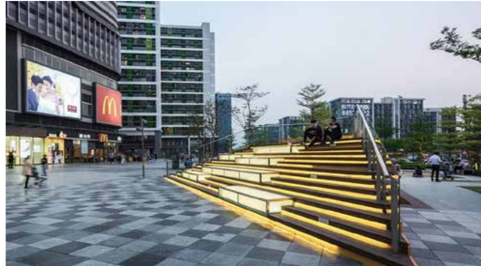
Figure 4.127 Example of lighting integrated into P3 bleachers
