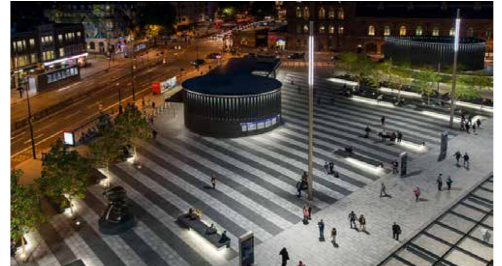
Figure 4.129 Pole mounted lighting to squares
