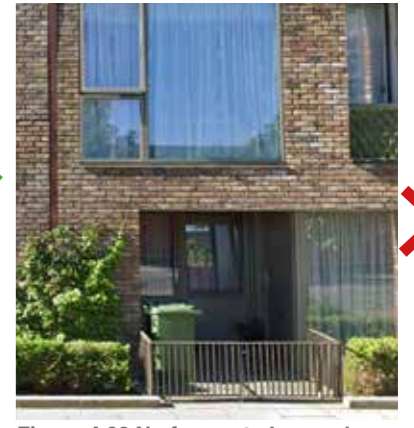
Figure 4.60 No fences to be used and no private space beyond the parcel limits. Bin storage to be integrated into architecture
