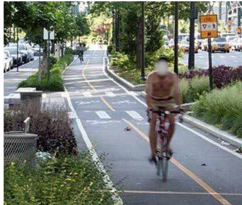
Figure 4.84 Planting used to separate the cyclist from pedestrians and vehicles
