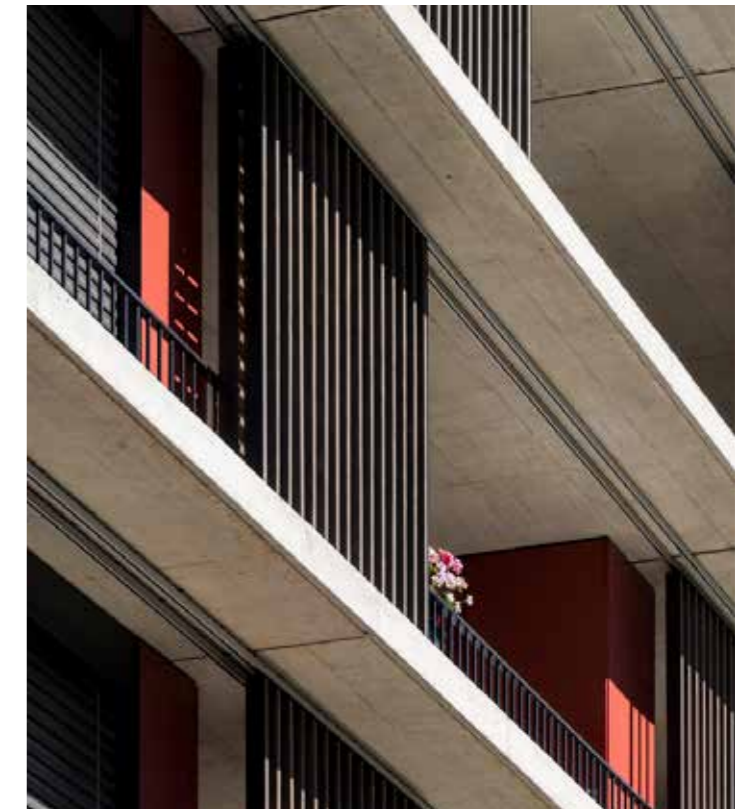
Figure 5.120 Example of screening design
