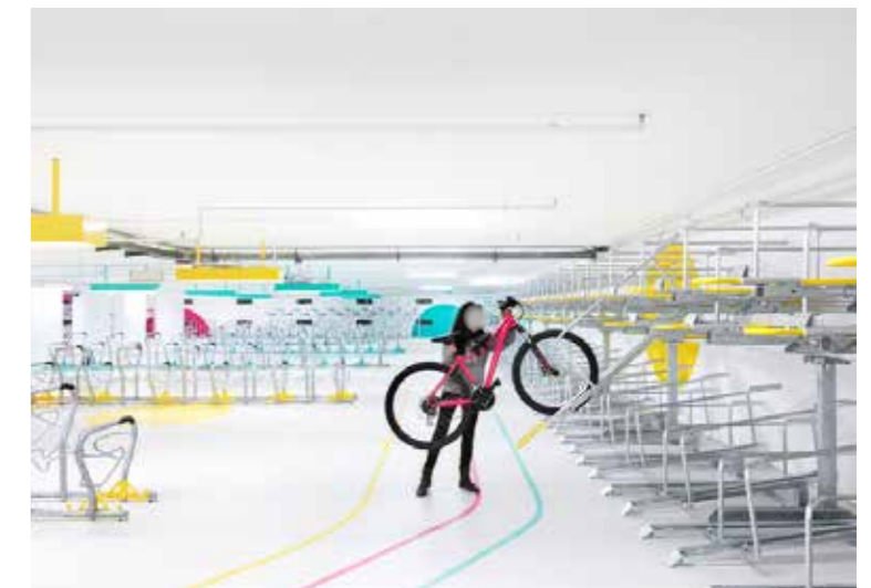
Figure 5.177 Bicycle storage system
