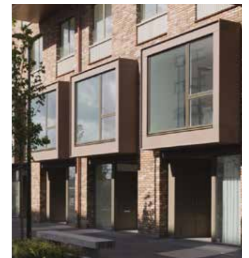
Figure 5.107 Example of an enclosed balcony /winter garden
