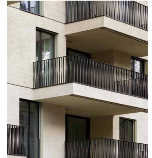
Figure 5.105 Example of projecting balcony
