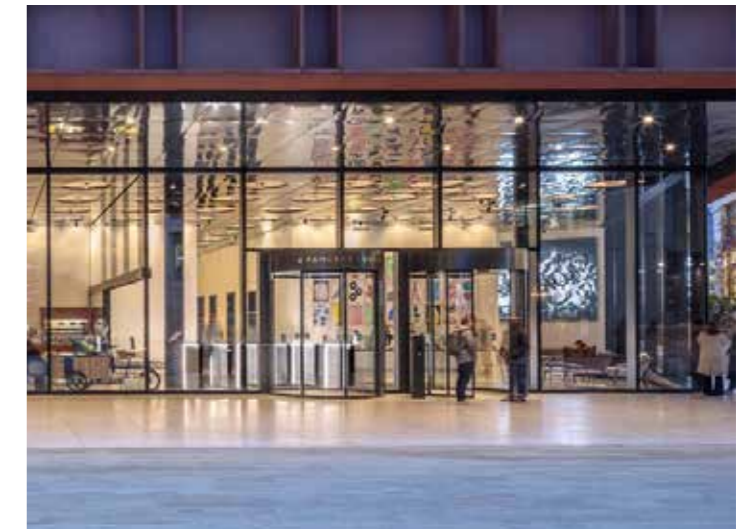
Figure 5.65 Commercial entrance integrated to façade
