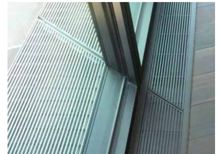
Figure 5.73 An example of a acceptable at ground level integrated vent - other through façade vents to follow similar levels of integration
