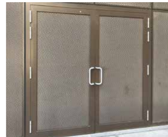
Figure 5.162 Example of detailing where ironmongery does not match overall material and tone compositions
