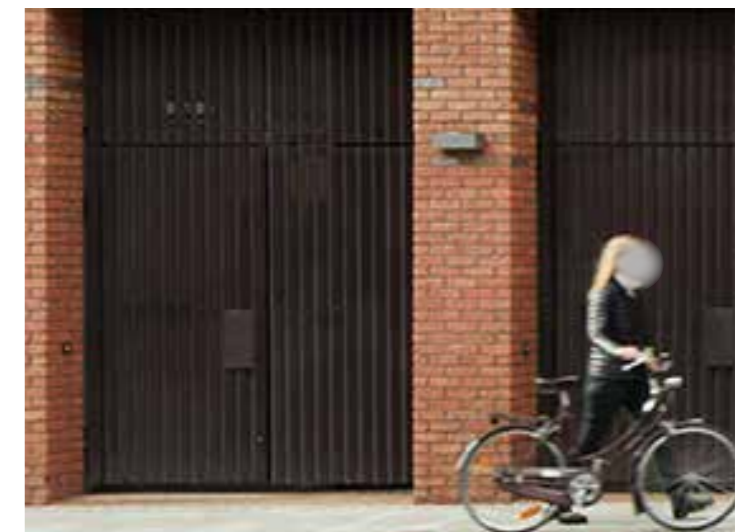
Figure 5.173 Screening in front of plant
