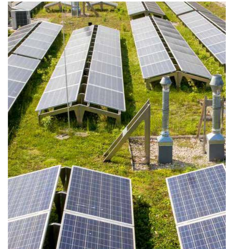
Figure 5.142 Opportunity for photovoltaic panels on the roof
