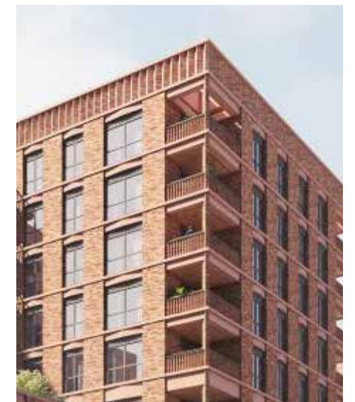
Figure 6.171 Example of inset balconies
