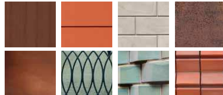
Figure 6.404 Various highlighting / detail material options of; acetylated or equivalent woods, terracotta, glazed tile/brick, weathered /anodised metals, general metalworking detail and texturing/relief of materials
