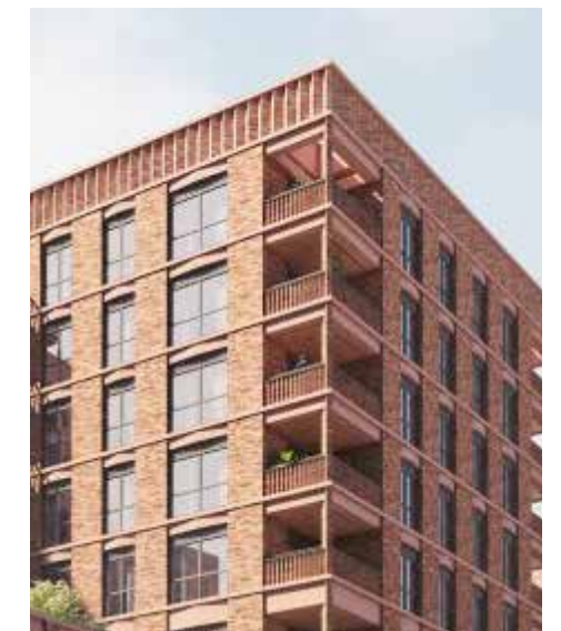
Figure 6.15 Example of inset balconies
