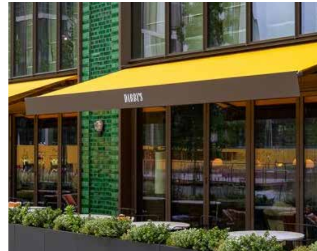
Figure 6.114 Example of awnings to retail
