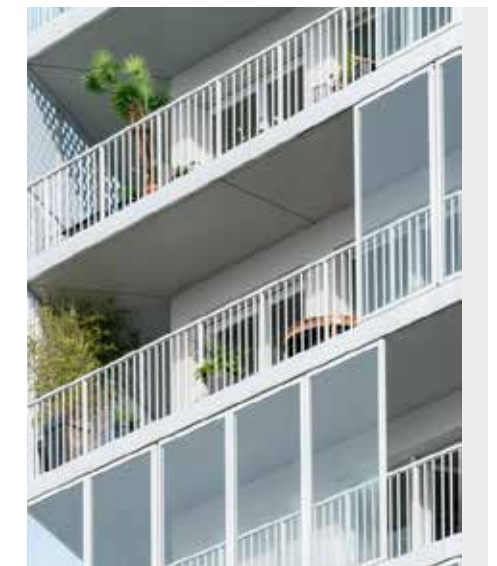
Figure 6.82 Example of inset balconies
