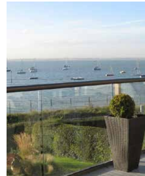
Figure 6.422 Example of 1.1m upstand
