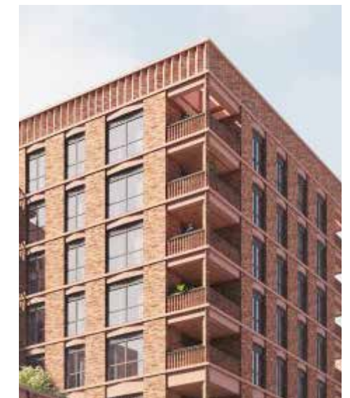
Figure 6.336 Example of inset balconies
