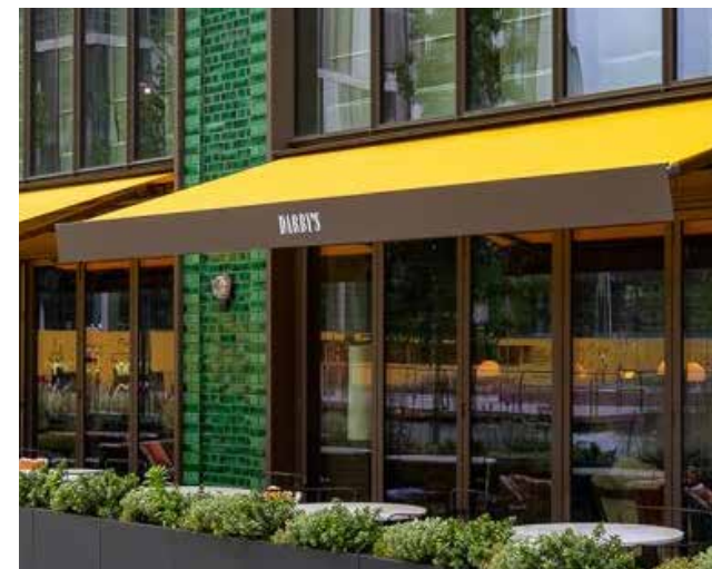
Figure 6.367 Example of awnings to retail
