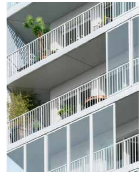
Figure 6.664 Example of inset balconies
