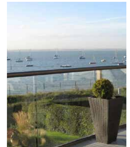
Figure 6.665 Example of 1.1m upstand
