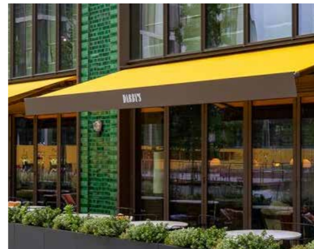
Figure 6.625 Example of awnings to retail
